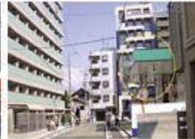
Station within Apartment Complex (Japan)
